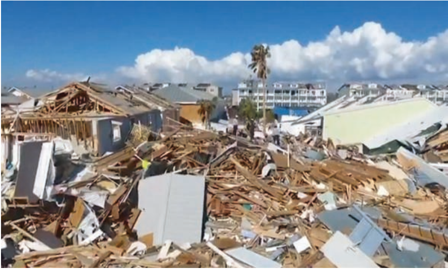
Fig. 8.2 Hurricane Michael damage. (Courtesy of Wikimedia Commons)
